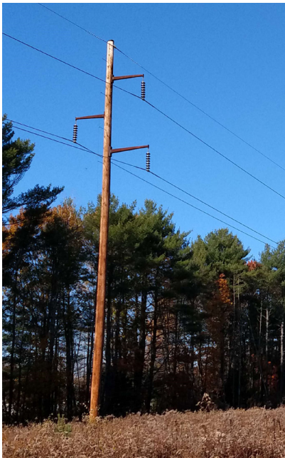
Type of pole being installed.
