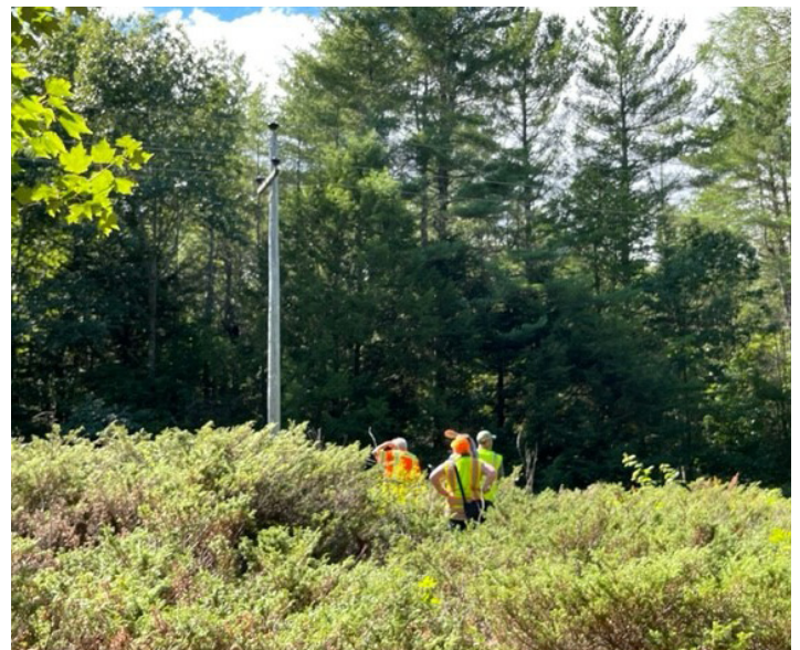
CMP Transmission Line Project Team members inspect one of the structures on Section 38 in Oakland.
